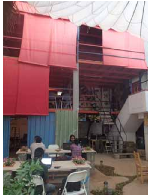
Jaaga building is built by pallet racks
